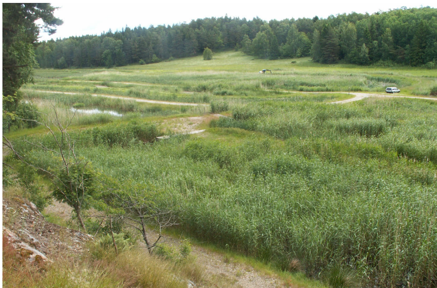
Figure 7.3 Wetland Alhagen with the first inlet wetlands and the alternately loaded West wetland (left), East wetland (background) and Inlet wetland (left of car) with bypass channel for stormwater between the pathways. Photo courtesy of Christer Svedin.
