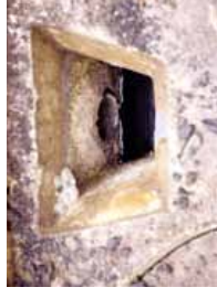
In this picture, looking down an outlet baffle, the effluent is below the pipe, indicating a bad seal.
