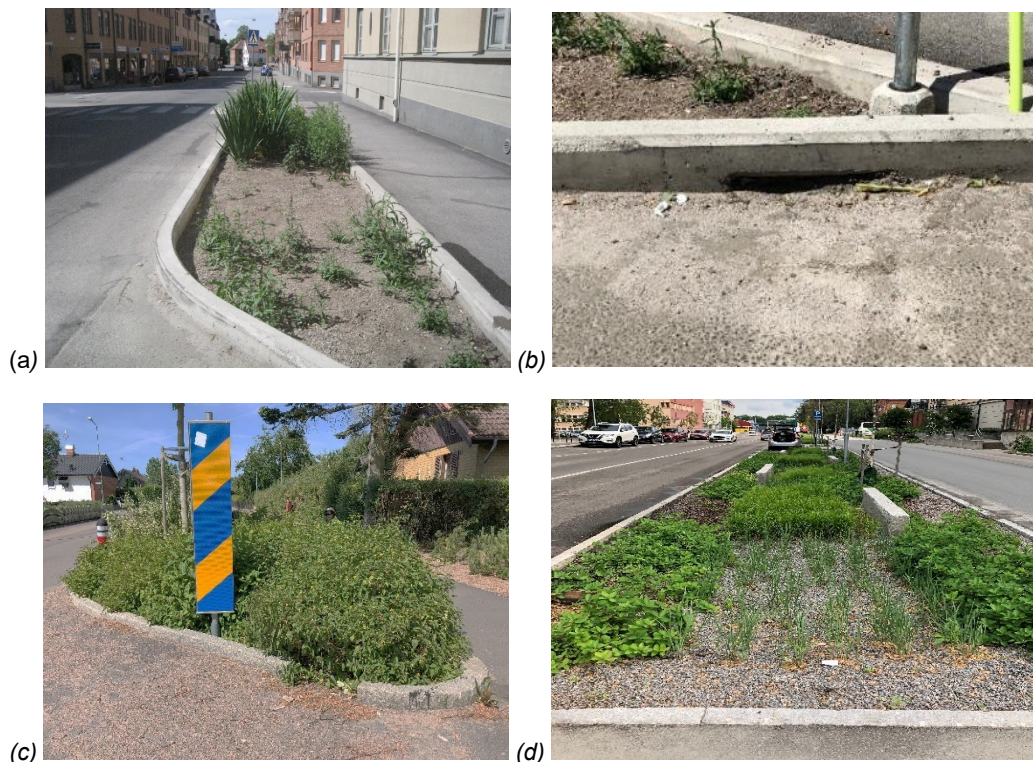
Figur 3. Vegetation i biofilter
