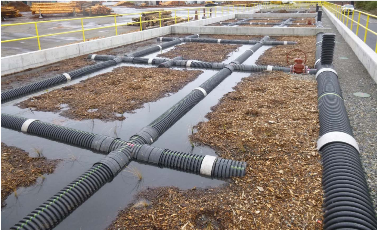
Figure 5 Post-construction: Stage 1 biofiltration distribution system in action.
